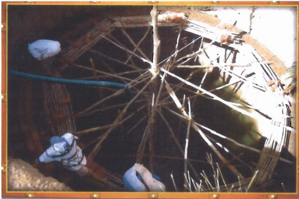
(strengthening of well at progress)
