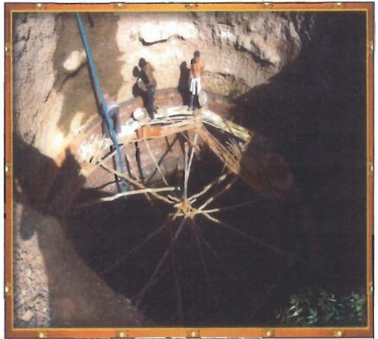
(NREGA well ,work site)
