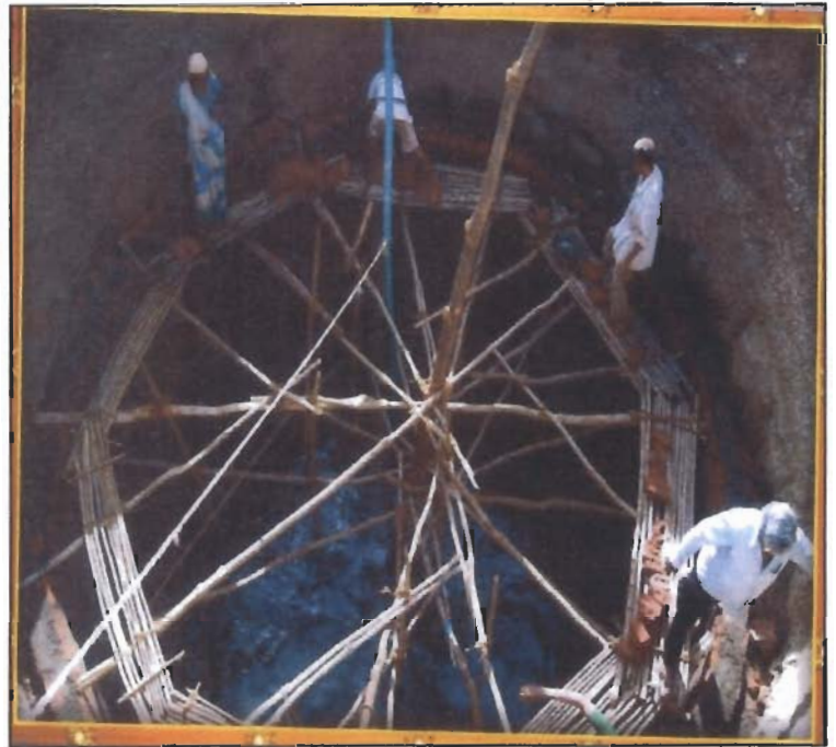
(NREGA well , work at progress)
